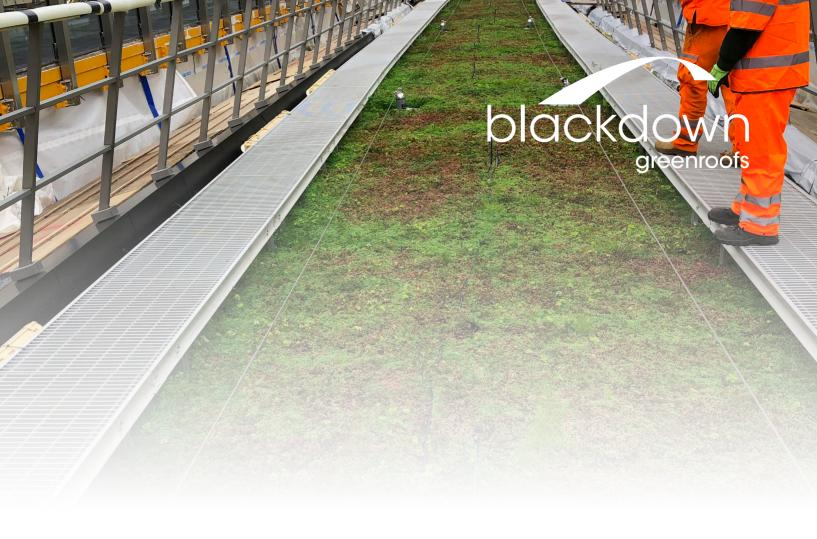
One of the main challenges with this project was that the station roof was curved from 0 to 22 degrees, which meant the green roof system had to be specially designed to function on a unique sloping surface. A specialised NatureMat® system was specified as it incorporated a 25mm fully wrapped drainage layer, a 50mm substrate and a 25mm sedum mat.
